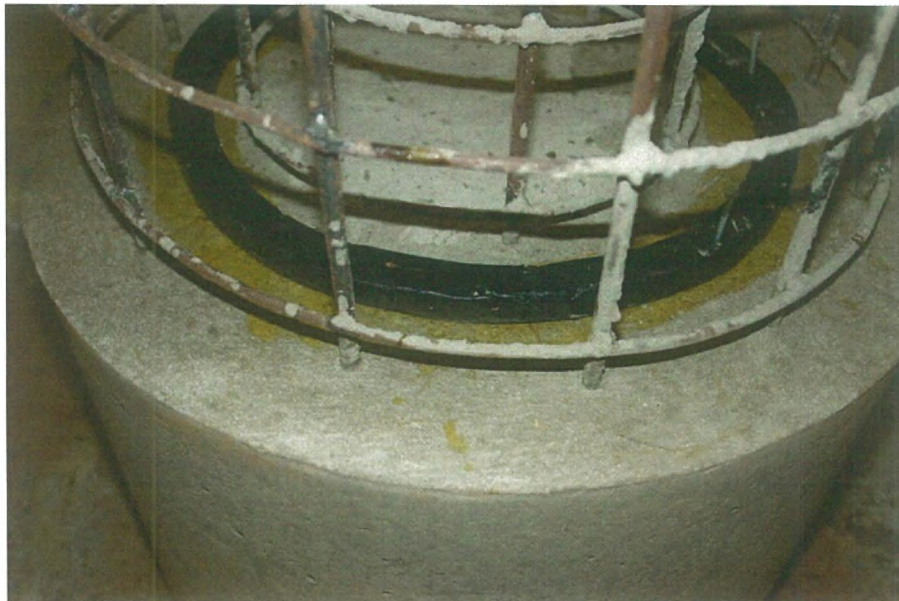
Photograph 2 - FERROSTOP 415 installed along the construction joint of the concrete test chamber.
